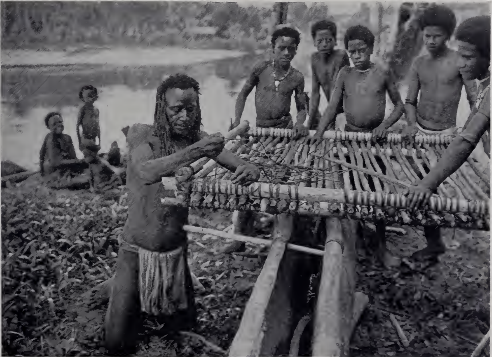
A Good Craftsman. Papuan builder making a boat deck. No nails are used, all the parts are held together with vegetable fibre string. Buildings capable of supporting the weight of hundreds of people are constructed in the same way.
